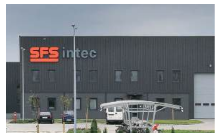
SFS Intec Kft., Jánossomorja - 12 pcs Hoval RoofVent® LW ventilation device
