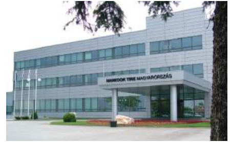
Hankook Tire, Rácalmás - 156 pcs Hoval RoofVent®, 47 pcs Hoval TopVent® TP units
