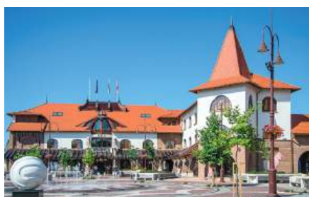
Mayor's office, Veresegyház - 3 pcs Hoval TopGas® gas condensing boilers
