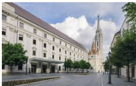
Hilton, Budapest - 3 pcs Hoval UltraGas® D gas boilers, 3 pcs Magnabosco rapid steam generator, eka chimney system
