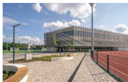
Dr. Koltai Jenő Sports center, Budapest - 10 pcs Hoval TopGas® gas condensing boilers
